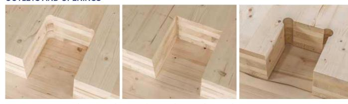
Whether you need recesses for purlins or rafters, outlets for heating / ventilation / sanitation facilities or window or door openings, an end mill can be used to design all kinds of outlets and openings. Corner cut-outs made with an end mill are usually round to begin with, but they can also be given sharp edges or milled diagonally.
