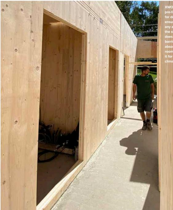
XWORKS buildings are fully pre-fabricated at the plant for dry assembly on site to ensure they do not transfer any additional moisture into the structure. The design does not include a diffusion barrier, so the walls can absorb the humidity in the room and evenly disperse it for a much nicer indoor climate.
