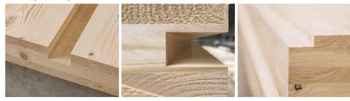
Full-length milling on the surface and front side as a rebate can be done with different thicknesses and depths, for example as a groove on the front side for a tongue on a separate piece.
